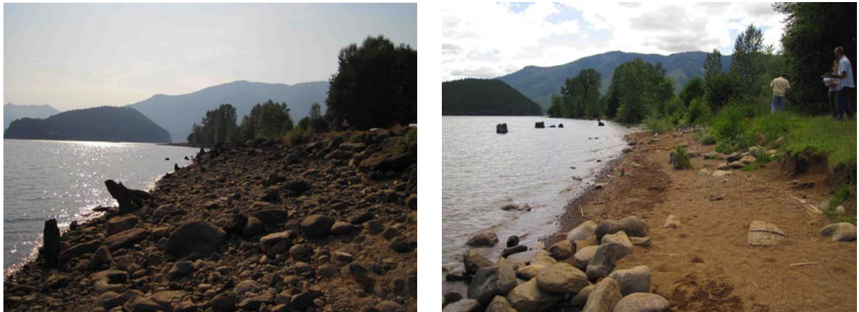
Fig. 7.5.4 - A,B; Detroit Flats Existing Shoreline Erosion
