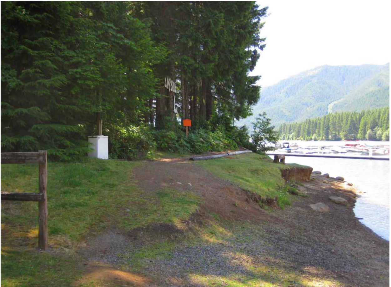
Fig. 6.5.2 - A; Kanes Marina Existing Trailhead
